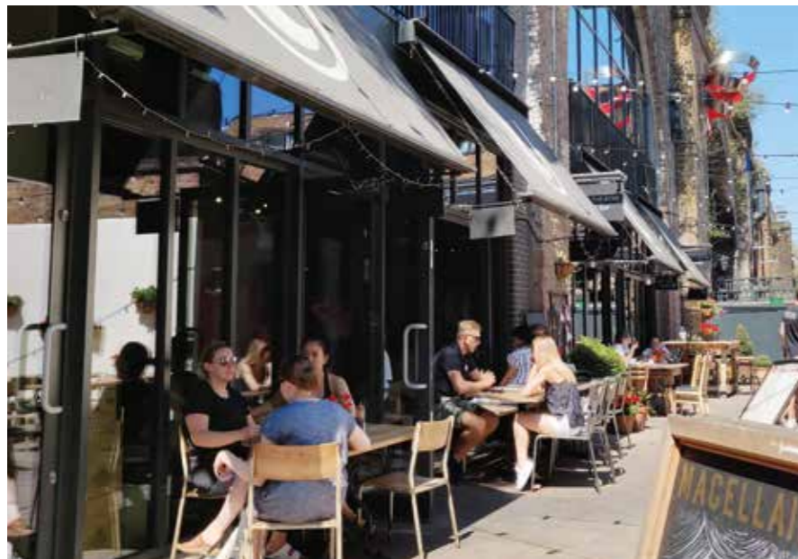
The reuse of railway arches will bring animation and character to the public realm
