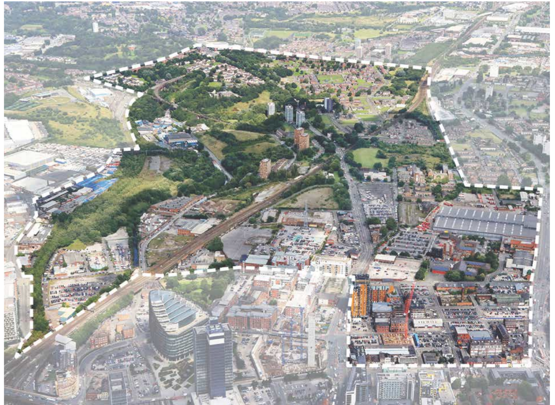
Figure 2 – Aerial view of the Northern Gateway
